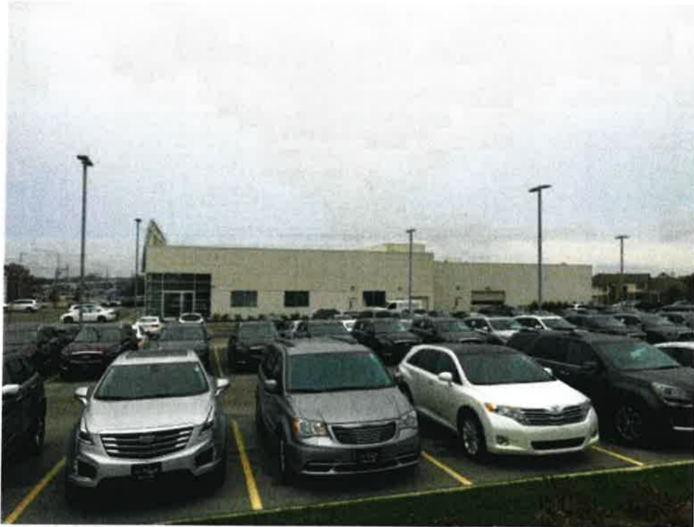
West Elevation – Side View of Subject Property
