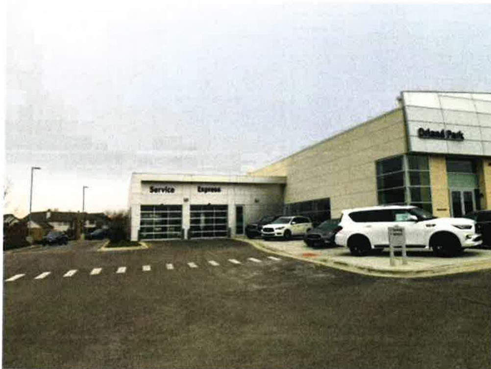
East Elevation – Side View of Subject Property
