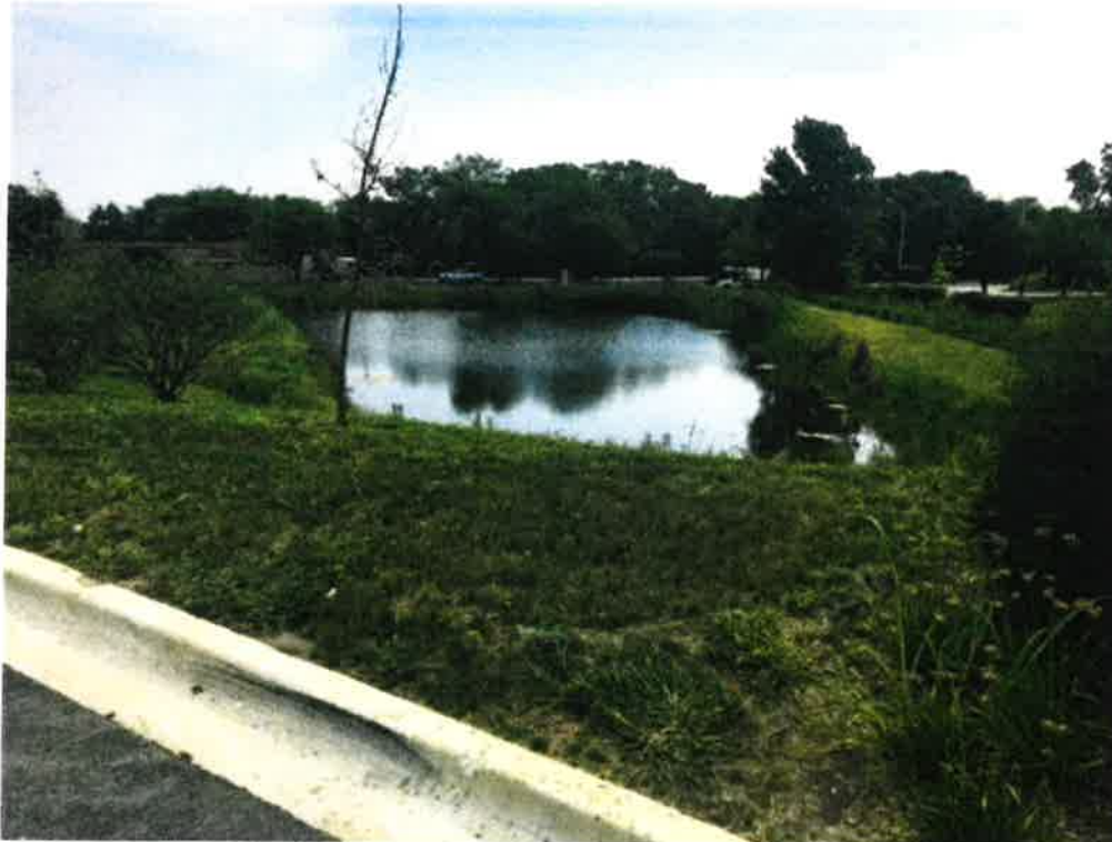
Retention Pond from 2018 inspection
