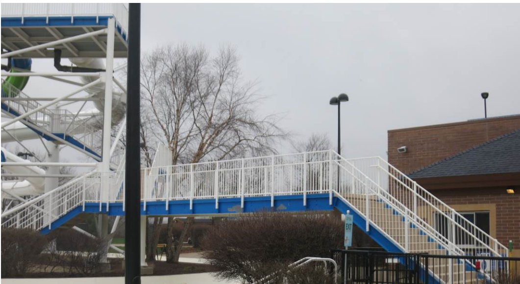
Photo No. 3 - Cross-walkway system to be investigated.
