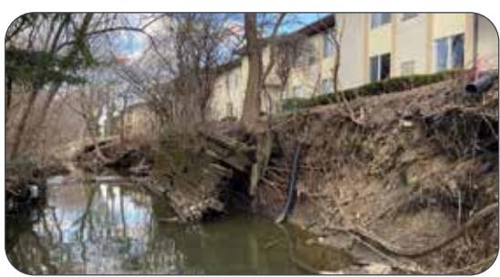
The proposed stabilization measures will address these concerns by reinforcing vulnerable bank sections, improving flow conveyance, and restoring the naturalized form and function of the stream.
