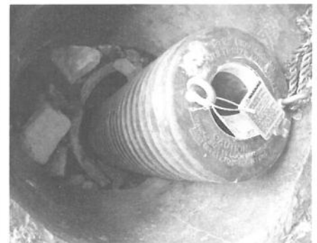
Pigging process for force main cleaning
