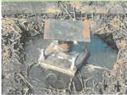
Installed Diamond Pier
