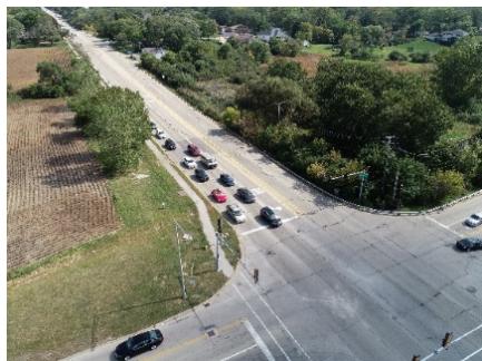
Looking West at the Dry Land Bridge
