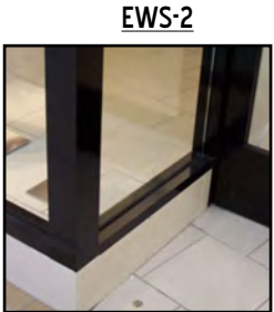
EWS-2 ALUMINUM STOREFRONT SYSTEM FINISH: ANODIZED BLACK
