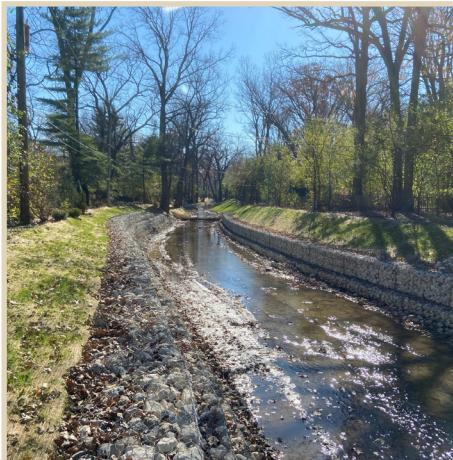
*V3 designed, permitted and constructed the streambank stabilization along two linear miles of the Skokie River in Lake Forest which included gabion walls, native vegetation, stone toe, bank reshaping, grading and drainage repairs.*
