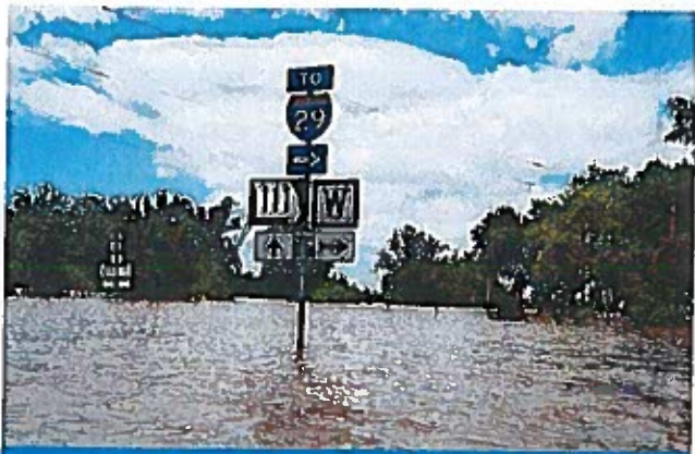
FLOOD AND WIND SENSORS INTEGRATION
