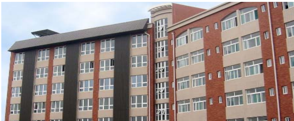
Above: Solar air heating systems attached to the façades of residential buildings. Light screening is recommended when facing public right-of-ways. Wall-mounted SAH units should face south for greatest exposure. Below: PV and SAH on a multi-family, mixed-use building.
