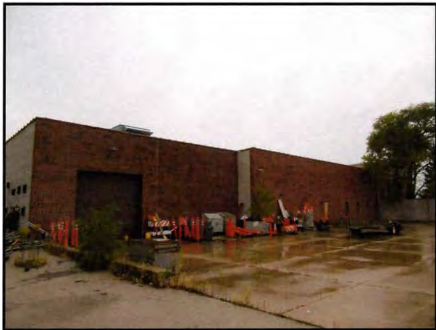
East Elevation of the Subject Property
