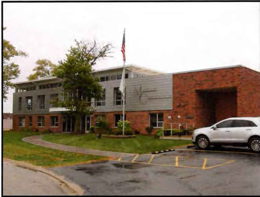
West Elevation of the Subject Property
