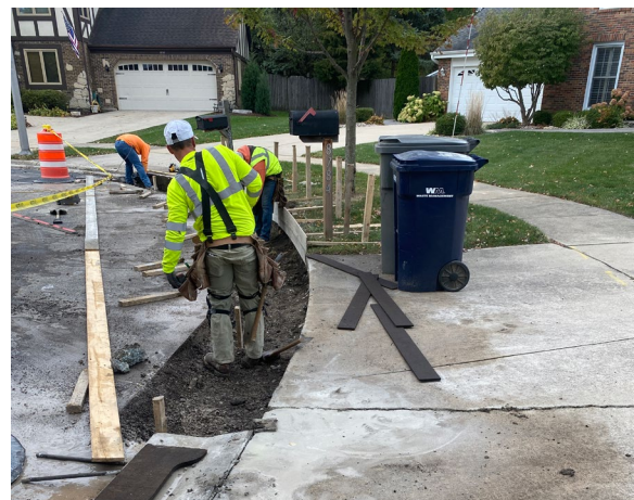
2020 Village Road Improvement Program
