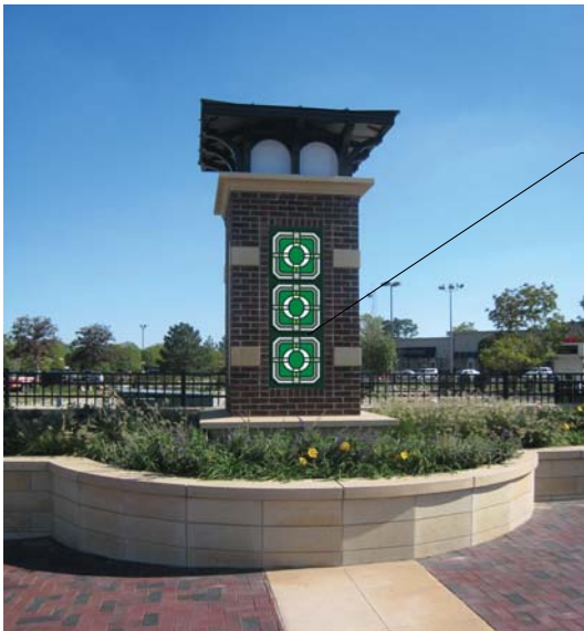
EX. PRIMARY MONUMENT RETROFIT (LaGrange/143rd)
