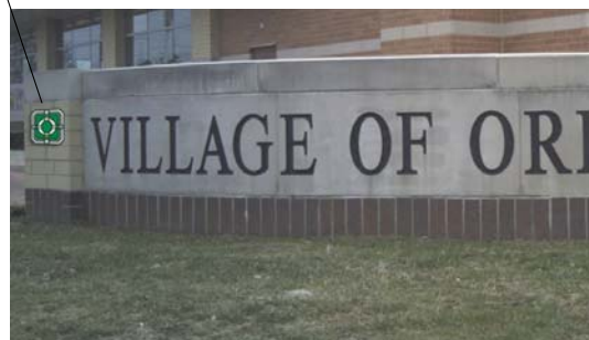
EX. GATEWAY MONUMENT RETROFIT (Will Cook/143rd)
