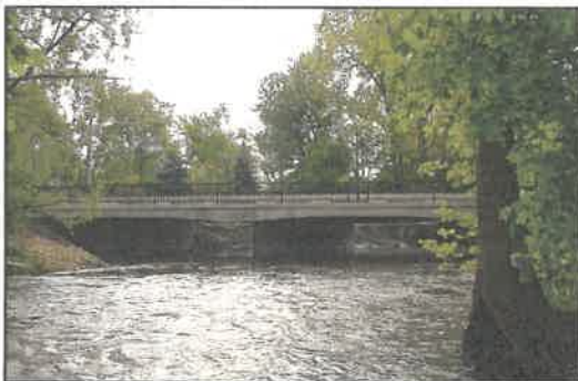
Hillside Road Bridge—Naperville, IL
