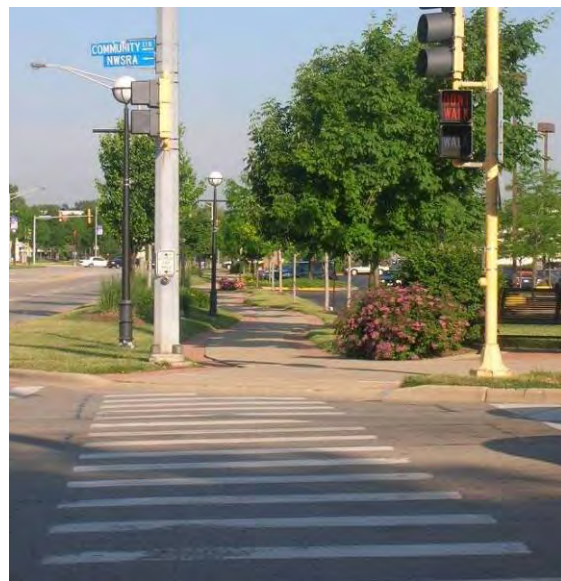
Pedestrian crossing with continental style pavement marking.
