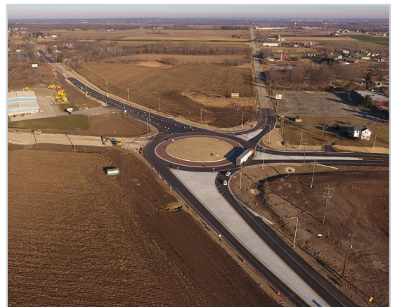
Drone footage of construction progress captured by Baxter & Woodman's in-house drone pilots
