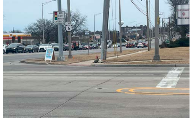
Figure 2. SE Corner. Highlighting no pedestrian accommodations or crosswalk.
