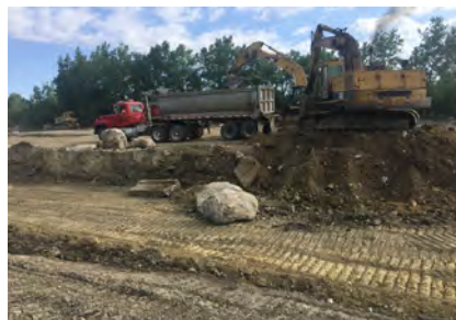
Construction of Veteran's Memorial Peninsula
