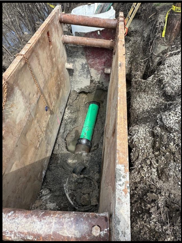
Southwest Highway Pipe Repair
