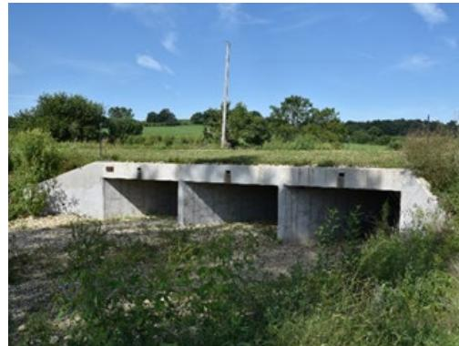
Box culvert was designed to better align with the stream to improve hydraulic and scour conditions.
