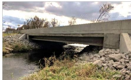
Single-span PPC I-Beam bridge replaced existing triple 60-inch CMP culverts.
