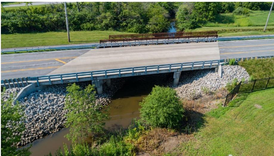
Three-span PPC deck beam bridge and pedestrian bridge over Union Creek in Frankfort, IL.
