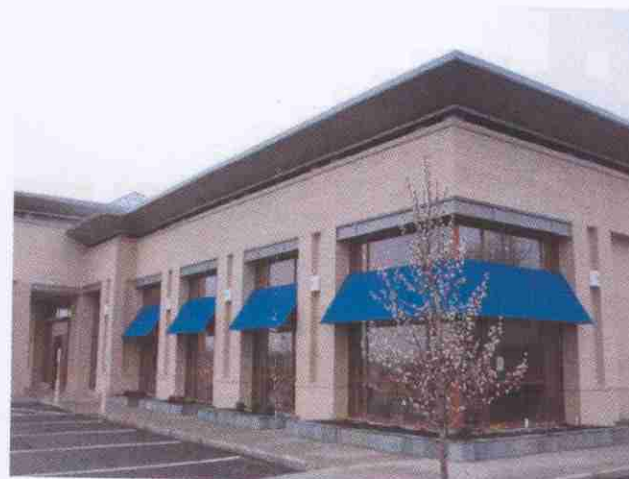
CORNER BUILDING DETAIL
