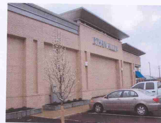
BACK BUILDING DETAIL
