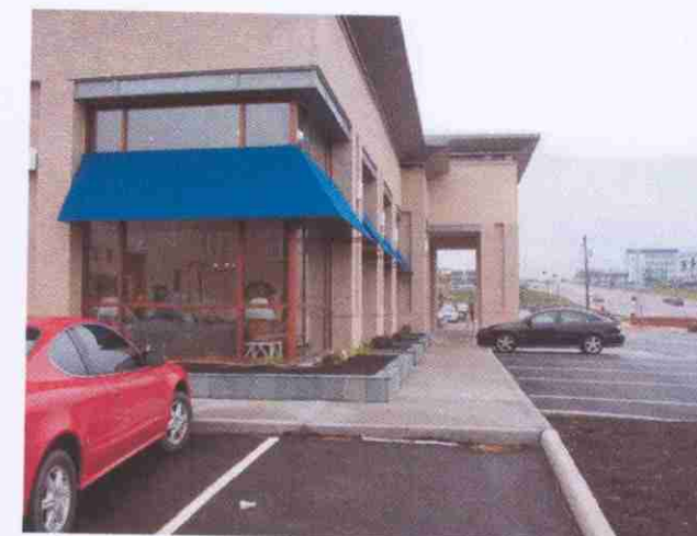
CORNER BUILDING DETAIL
