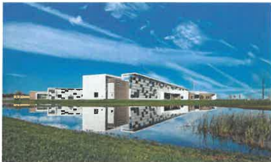
Illinois National Guard Readiness Center and Army Aviation Support Facility
