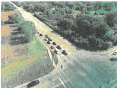
Looking West at the Dry Land Bridge
