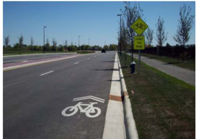
Wide outside lane with sharrows and "Share the Road" sign. Sidepath also provided for less experienced riders.
