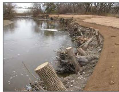
Image: post-construction crib-wall, pre, pre-vegetation.
