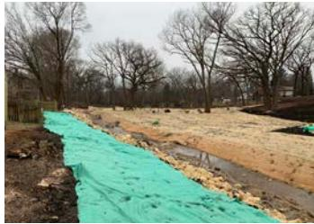
► Example of turf seeded area with netless blanket to the top of slope
