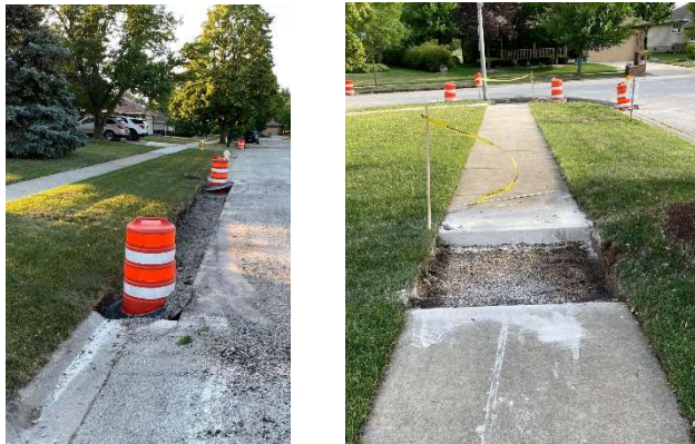
Before: Drums installed along curbs
