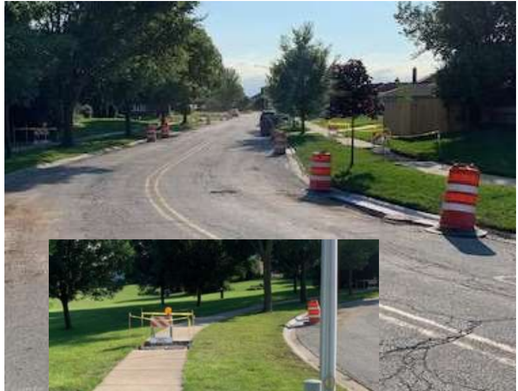
After: Type II Barriers installed at sidewalk
