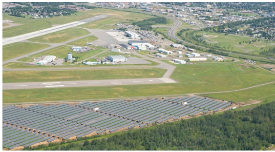
The 8.5MW Thunder Bay Airport Solar Park (Image via Recharge News .)
