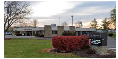
Police Department Renovation Village of Shorewood
