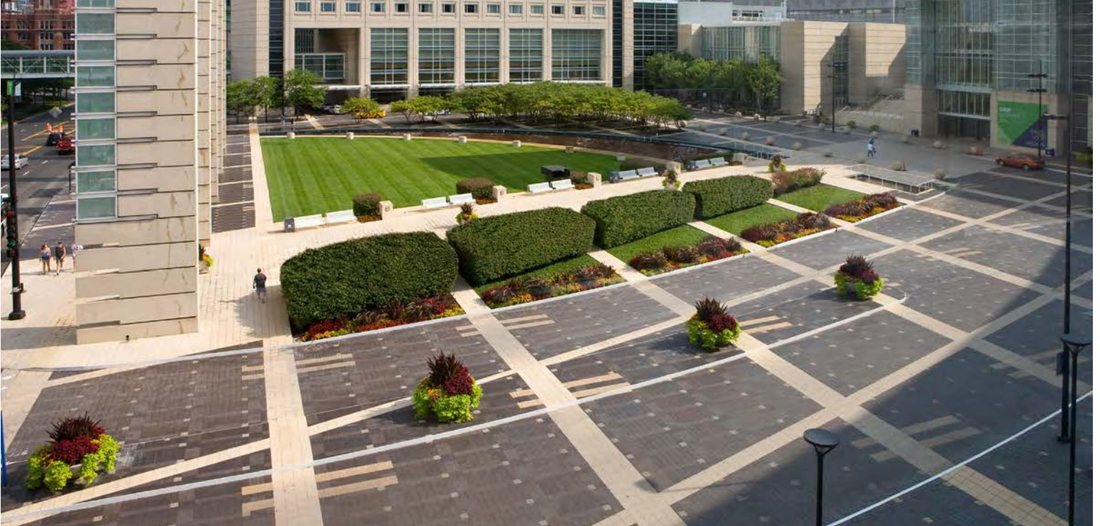
McCORMICK PLACE FRONT ENTRANCE
