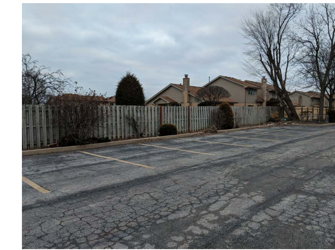
6' TALL EXISTING FENCE VIEW FROM PROJECT SITE
