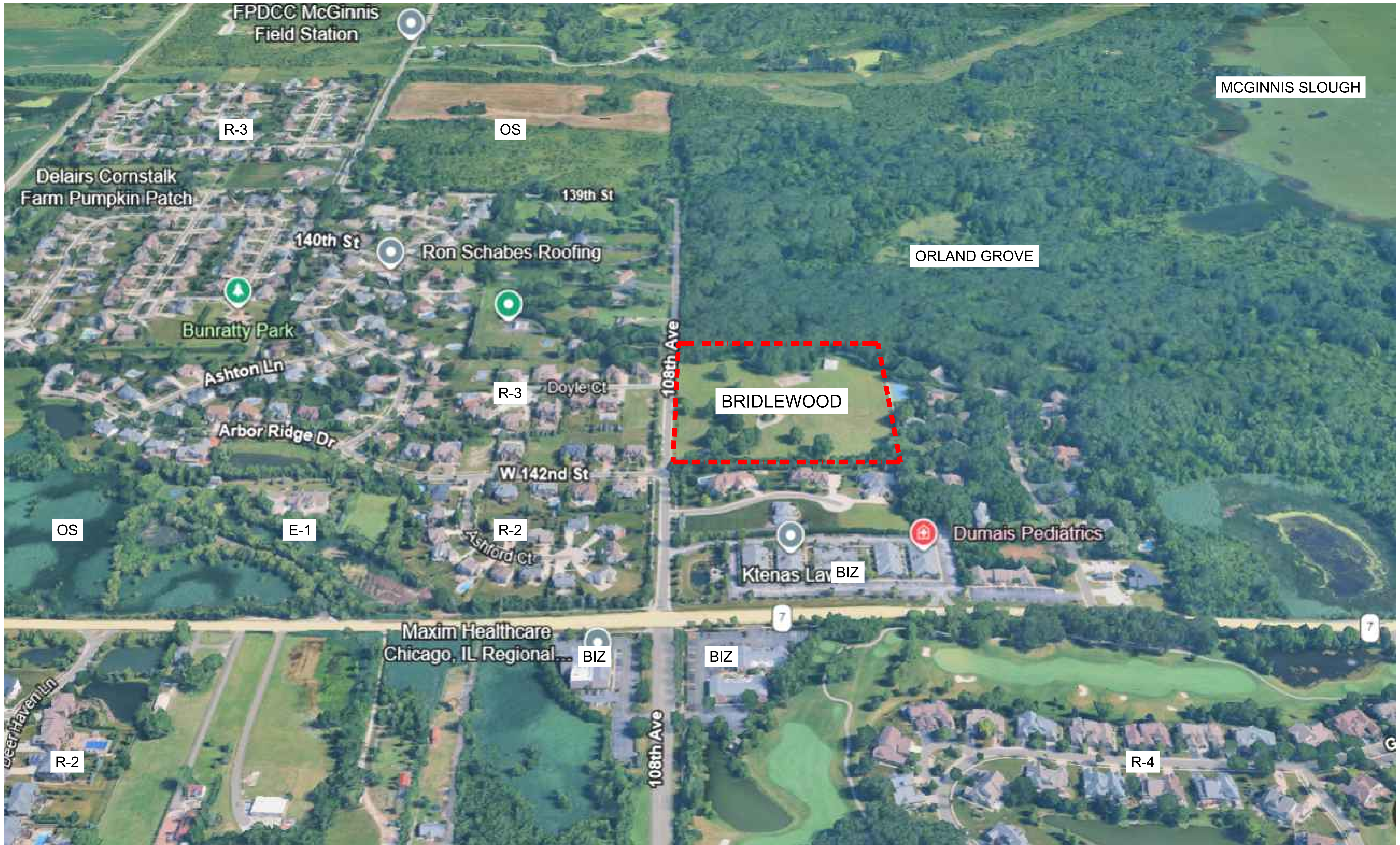
AERIAL OF SITE VIEWING NORTH
