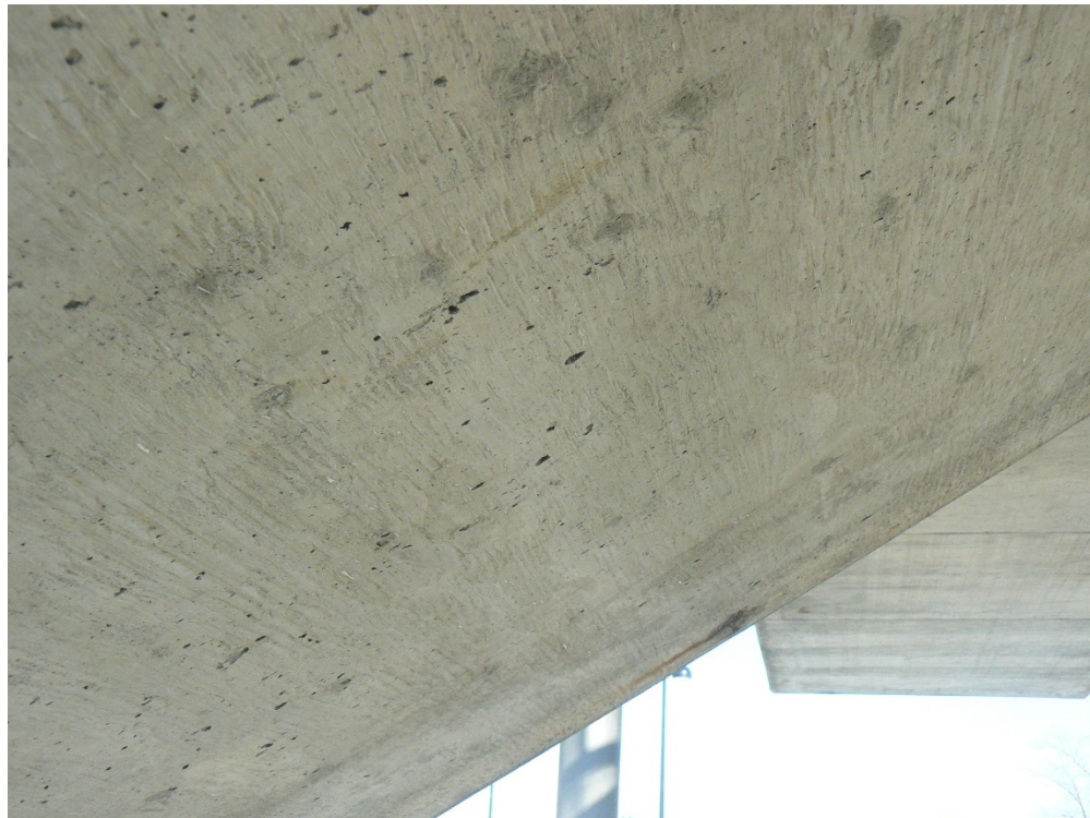
Crack I - underside of stairs – hairline crack, probably too small to inject at this time
