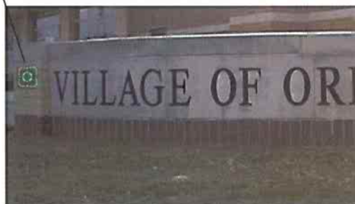
EX. GATEWAY MONUMENT RETROFIT (Will Cook/143rd)
