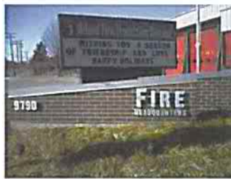
Fire Station 1 (Retrofit)
