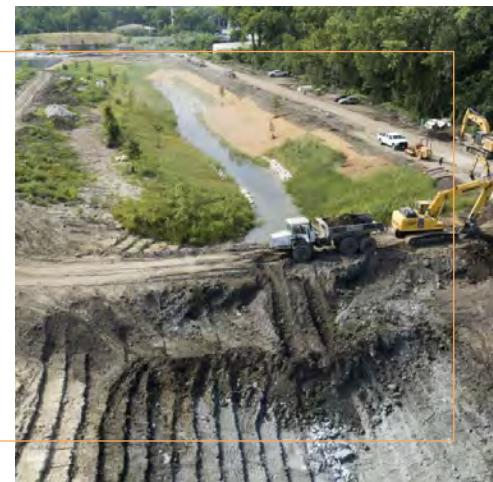
**Lacey Creek Emergency Bank Stabilization • Downers Grove Sanitary District** • Protecting a 24-inch sanitary sewer forcemain adjacent to eroding creek banks required immediate stabilization measures. We designed and permitted structural improvements along 117 feet of Lacey Creek, delivering a fast-tracked solution that met regulatory requirements and ensured long-term protection for critical infrastructure.
