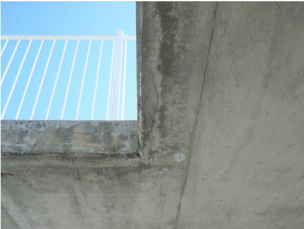
Crack D – Underside of main platform
