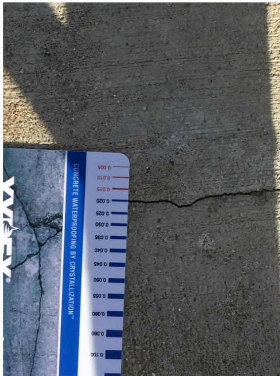
Close-up of crack A on top slab – measured 0.020"
