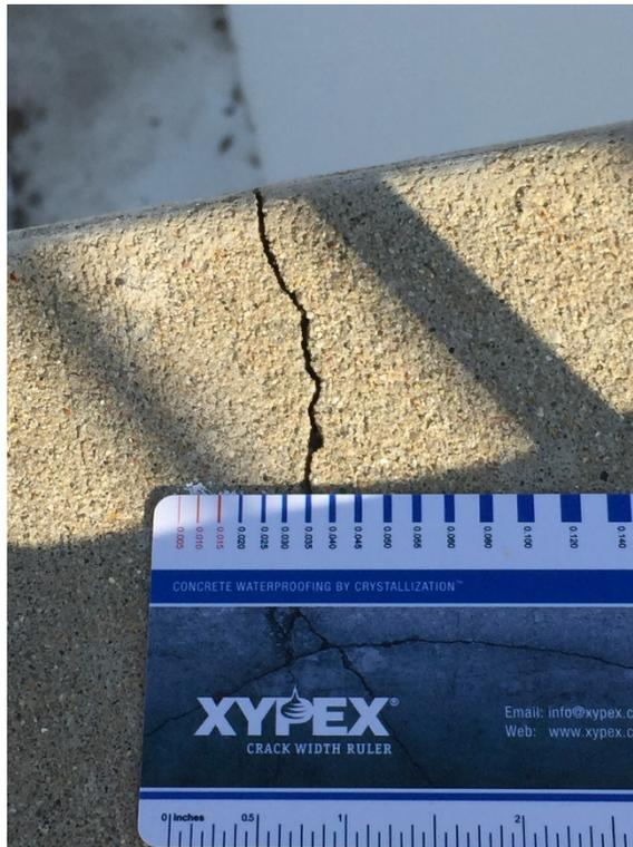
Close-up of crack E on top slab – measured 0.035"
