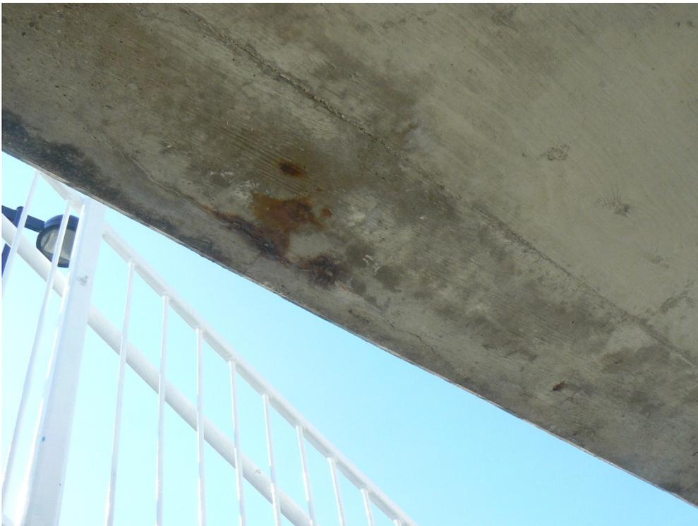
Crack G – Underside of main platform – with minor rust and efflorescence
