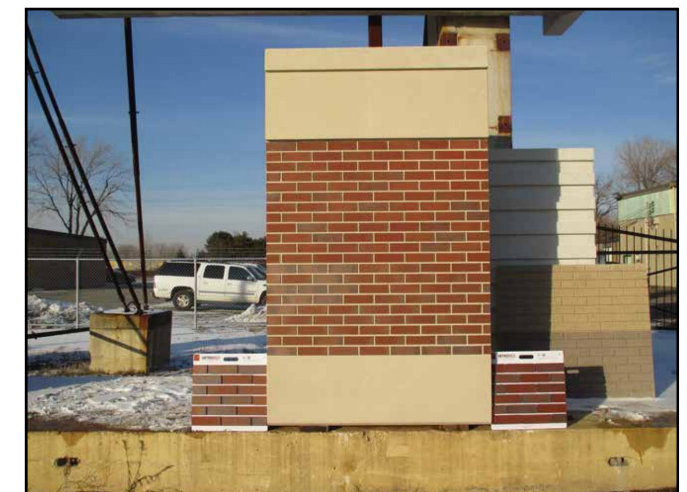
PHOTOGRAPH OF ACTUAL BRICK & PRECAST MOCK-UP
