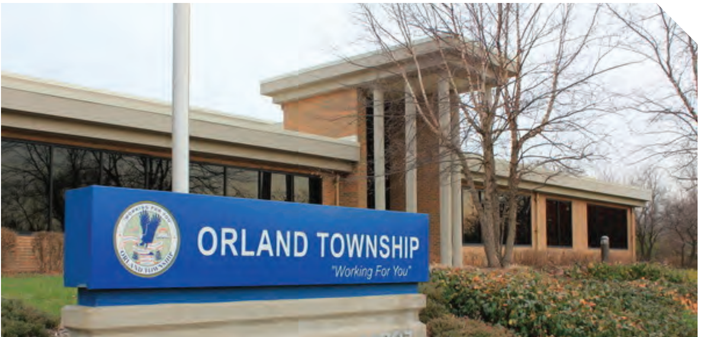
Figure 7: Orland Township Building
