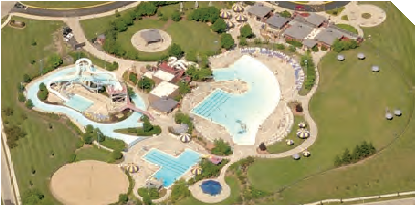
Figure 6: Centennial Park Aquatic Center
