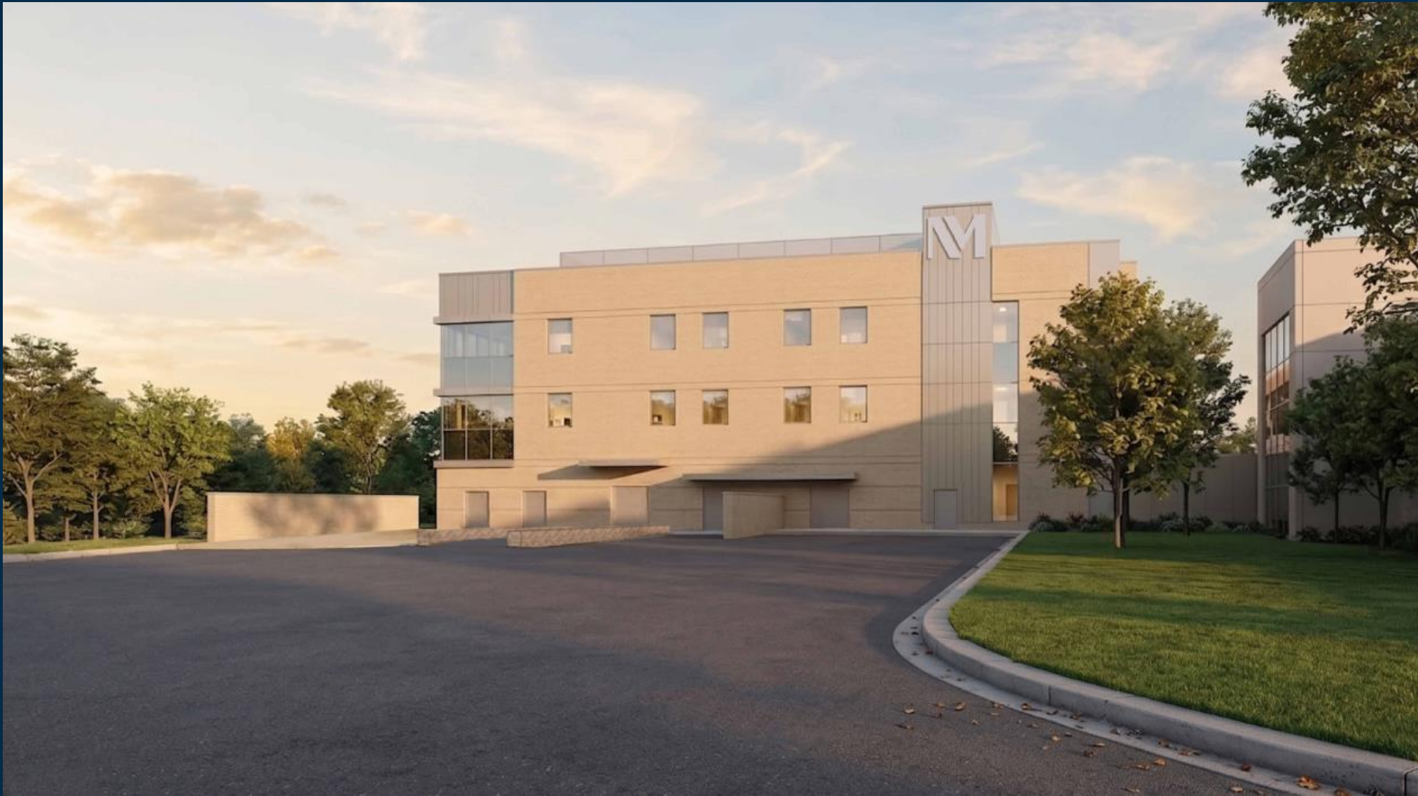
LOADING DOCK AND AMBULANCE – WEST FACADE
