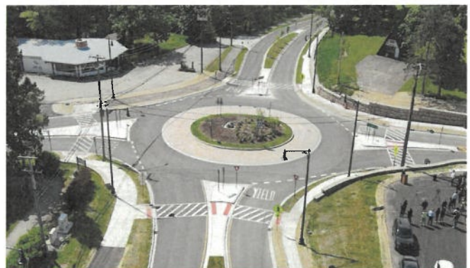
Algonquin Main Street Reconstruction Project
