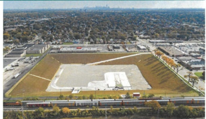
MWRDGC Addison Creek Reservoir Project
