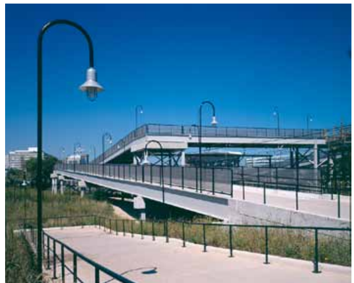
18th Street Pedestrian Bridge
