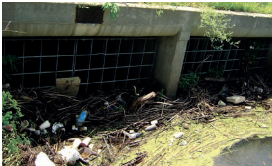
Trash and Debris Accumulation and Channel Modification, Frankfort Tributary
