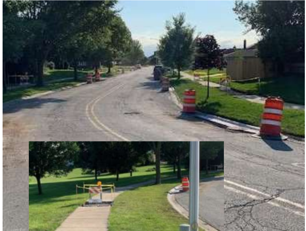
After: Type II Barriers installed at sidewalk
