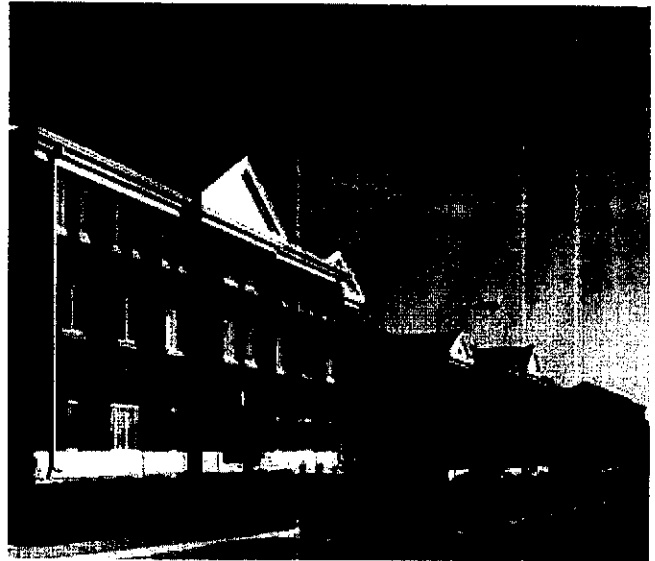
MCPON Plackett Manor Bachelor Enlisted Quarters
