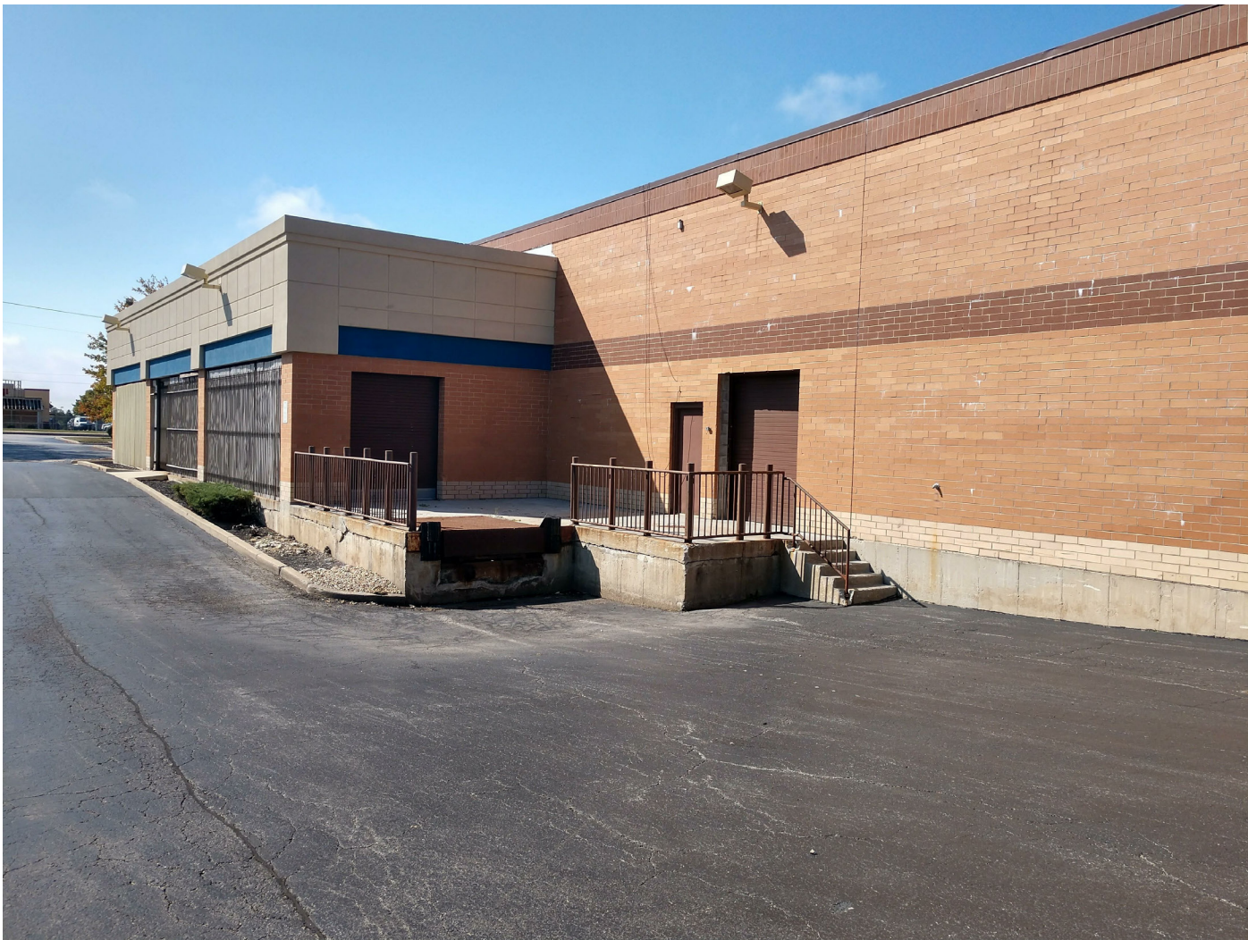
EXISTING CONDITIONS (DOCK AREA, LOOKING SOUTHWEST)
