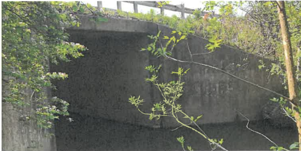
Existing structure under 82nd Avenue at Tinley Creek
