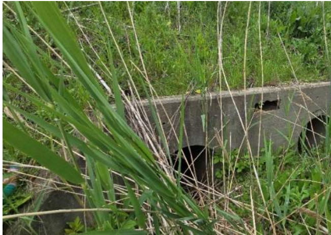
Photo 5: From SP-13, view of culvert and Wetland 4
