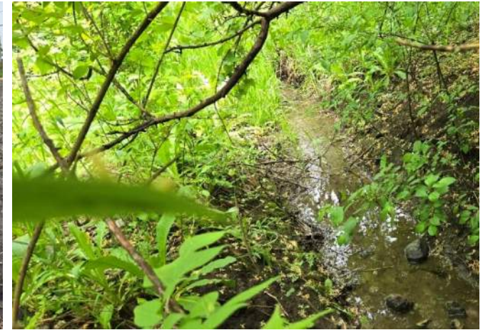
Photo 9: View of Southern Culvert
