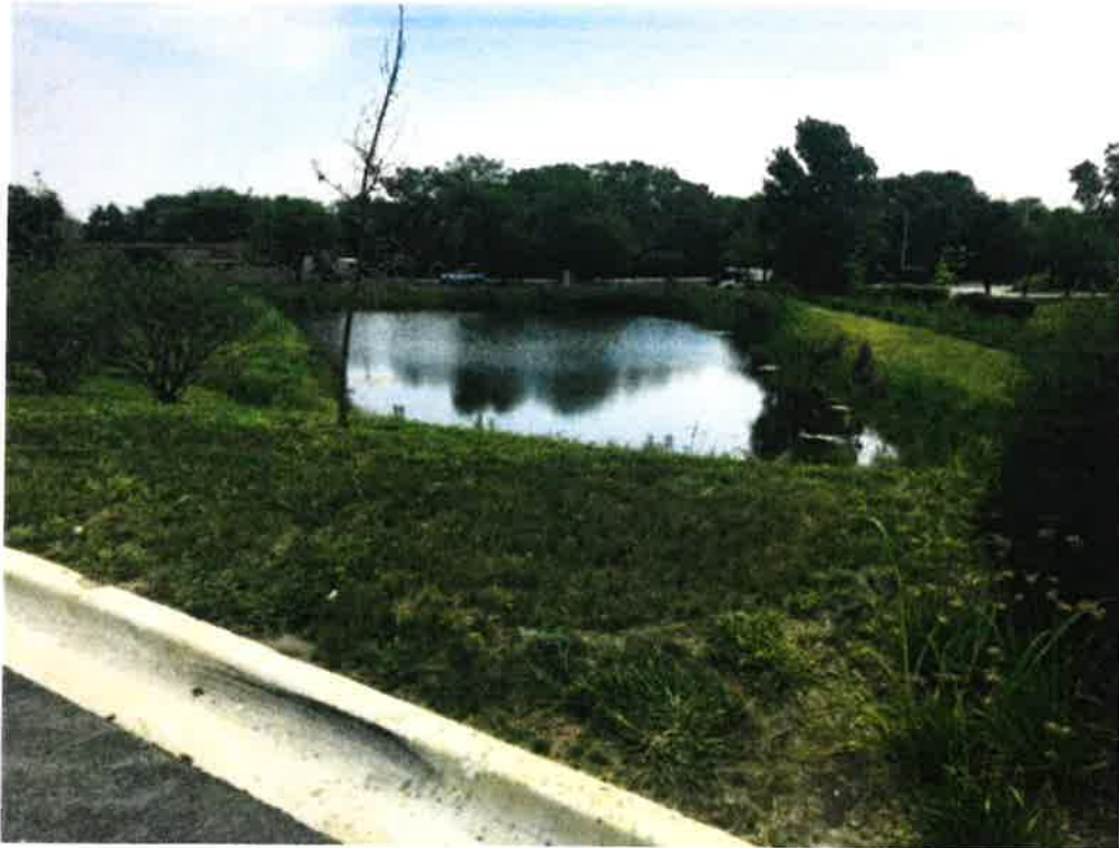
Retention Pond from 2018 inspection
