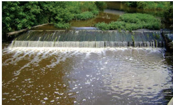
Spring Creek Dam at Draper Avenue, Joliet
