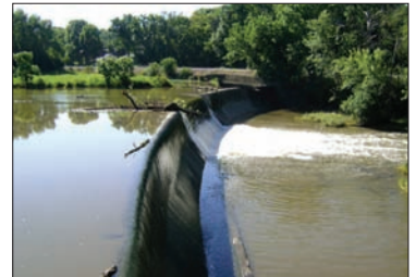
Dam on Hickory Creek at Pilcher Park
