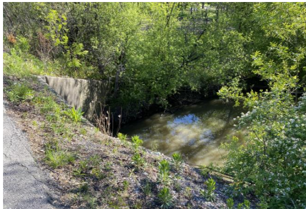
Box culvert carrying Tinley Creek under 82 nd Avenue.
