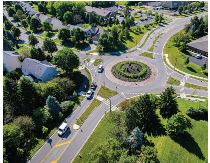
Snider Road and Thornberry Court roundabout.
