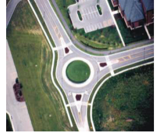
Aerial view of Navajo Drive roundabout.
